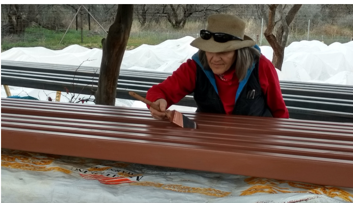
Gail priming and painting the steel frame
