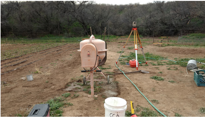
February 2019: Clearing the site
