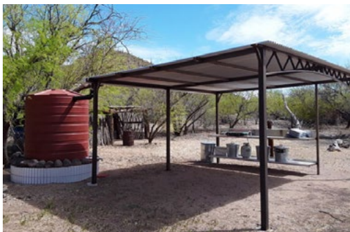
New rainwater catchment system at the Corbett Center doubles as a shade ramada
